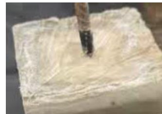
Figure 1. Example of steel reinforcement embedded in the concrete, after accelerated corrosion testing.
