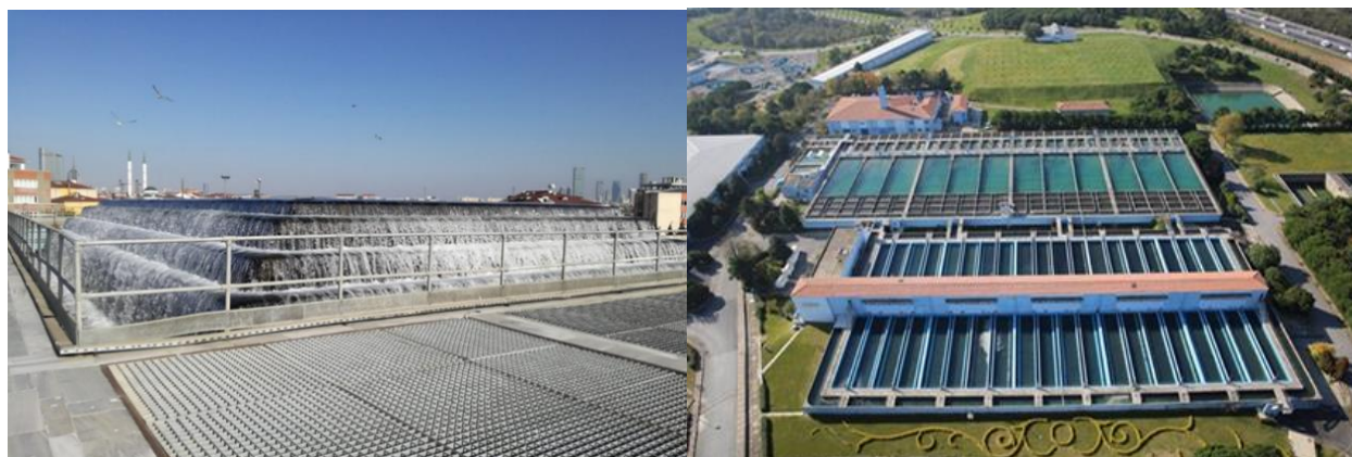
Figure 2. Aeration unit and rapid sand filters
