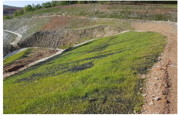
Figure 4. Hydroseeding results earthen slope with synthetic geotextile and in after 3 months in R.D. of Chalkidiki. Semi-rocky slope with synthetic geotextile
