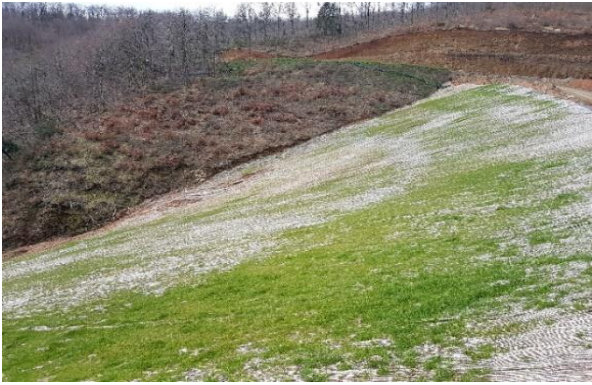
Figure 3. Hydroseeding results earthen slope with organic geotextile after 3 months in R.D. of Chalkidiki. Earthen slope with organic geotextile and in the right image a semi-rocky slope with synthetic geotextile
